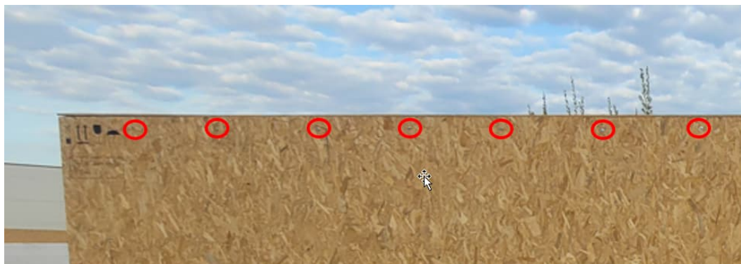
Fig. 7: Screws of the cover timbers
